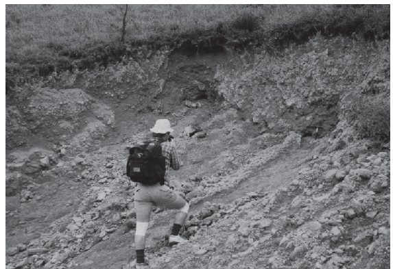
Figure 10. Failure involving surface mantle of colluvium
